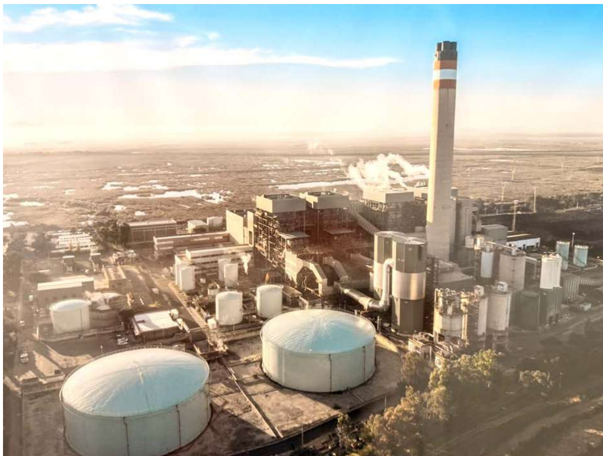
Figure 1: aerial view of the plant. On the left side is unit 1&2 and on the right side 3&4
