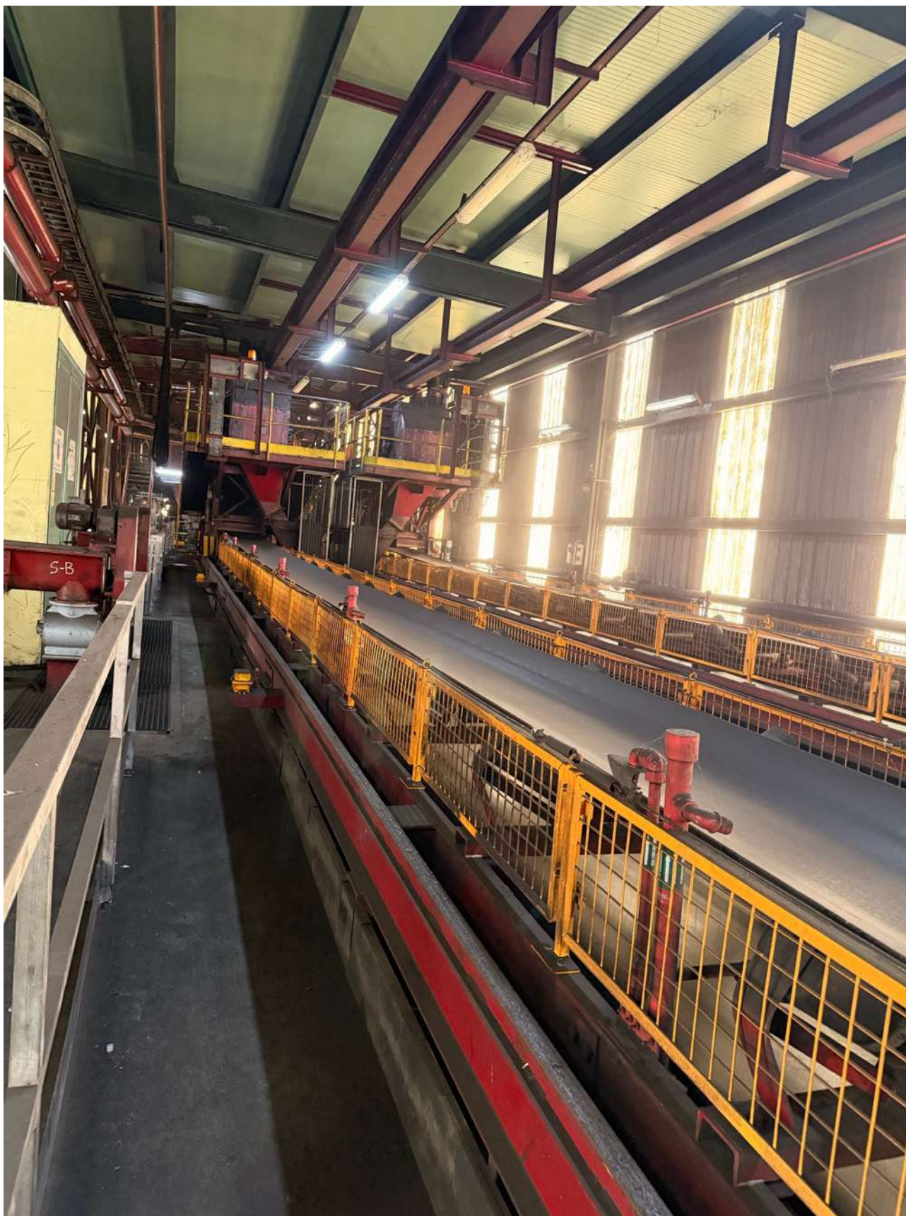
Figure 25: coal conveyor building.
