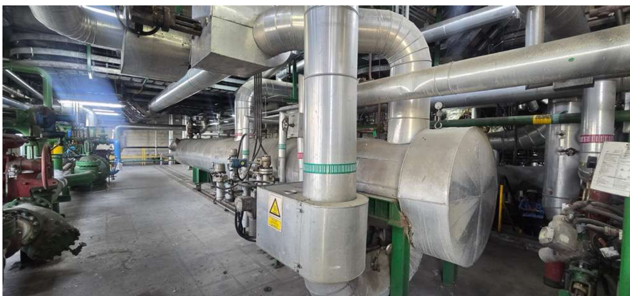
Figure 8: detail preheaters. All are visually in perfect condition.
